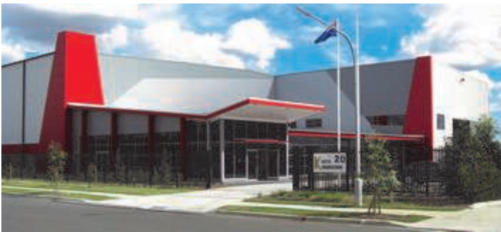
Keith Engineering's new premises at Erskine Park
