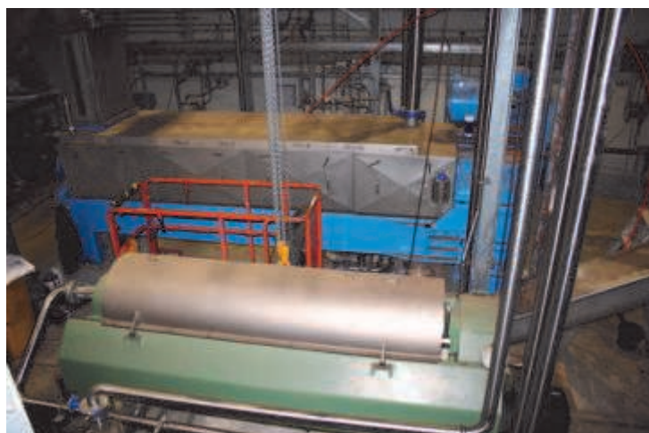
Twin screw press and decanter being installed at Talloman
