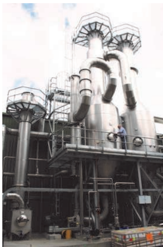
Andy Bennett conducts maintenance on the new evaporators
